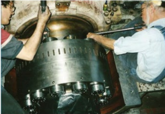
Superbolt replacements for 12 fitted studs on a 400-MW steam turbine: 12 EzFit mechanical expansion bolts, each secured by two multi-jackbolt tensioners. Torque required was only 55 ft-lb
